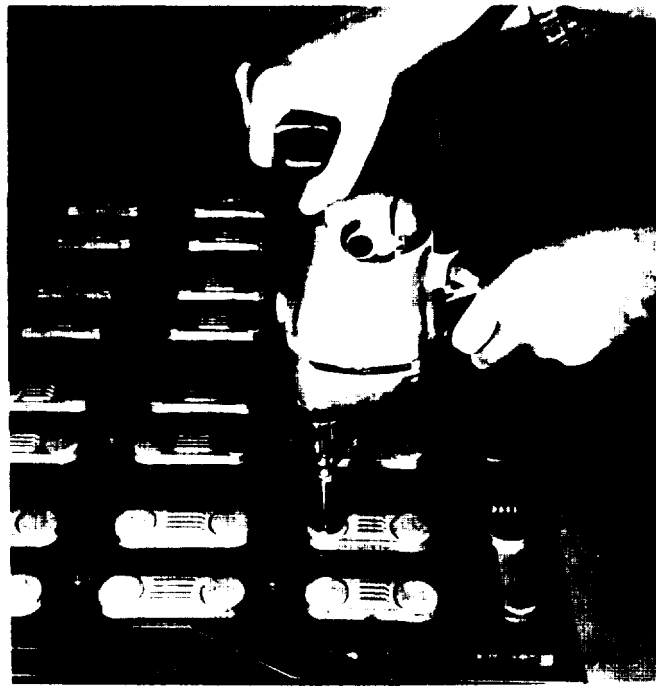
Figure 3-1. Drilling cell connector
