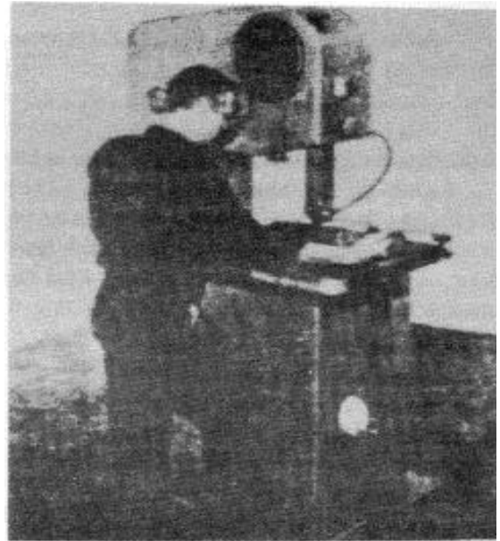
Fig. 21. Set the weight for the power feed by pressing down on the foot pedal.
