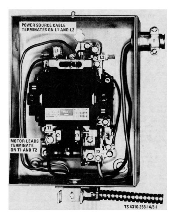
Figure 5-1. Magnetic starter (shown with cover removed).
