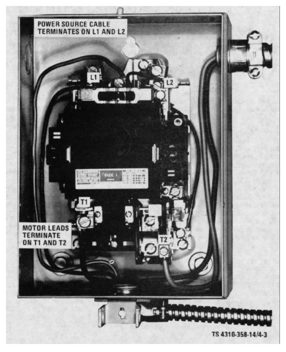
Figure 4-3. Magnetic starter (shown with cover removed).
